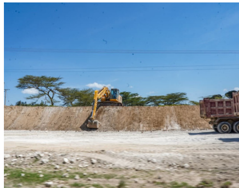
A section of Rironi-Mau Summit road works
