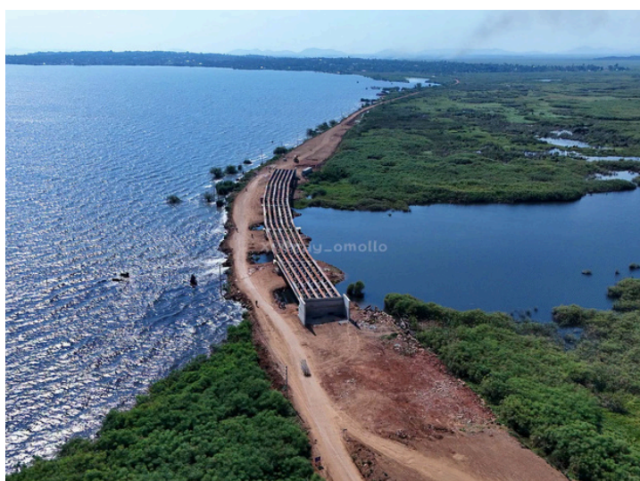
Construction of the strategic 200-metre Composite Steel Girder Dhogoye Bridge in Usenge recorded notable progress. Once completed, the bridge will permanently restore a vital transport link along the Kisian-Usenge-Osieko Road corridor.
