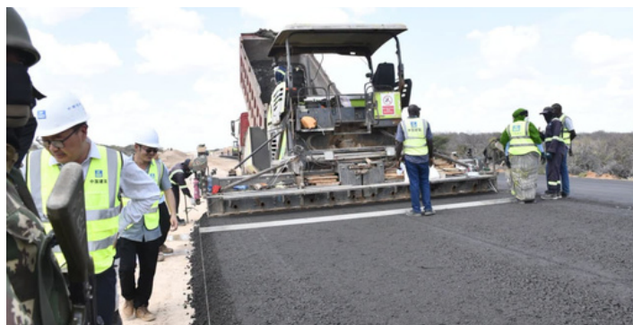
Ongoing construction works along the Isiolo–Kulamawe–Modogashe–Wajir road corridor during an assessment by the HoAGDP Implementation Support Mission on 9 th June, 2026.
