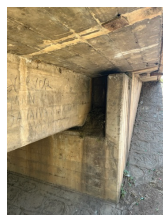
Siltation/Sedimentation on the bridge seat.
