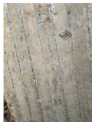
Cracks on the deck slab.
