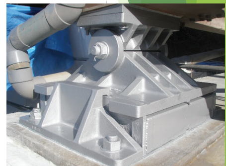
Sprayed steel bearing
