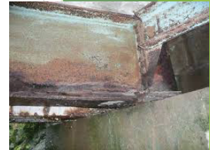
Corrosion of steel girder.
