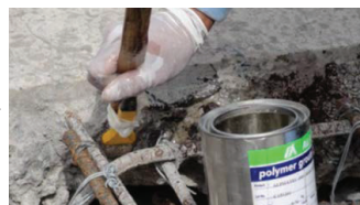
Applying epoxy bonding material.
