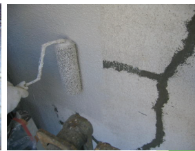
Cut & Fill work
