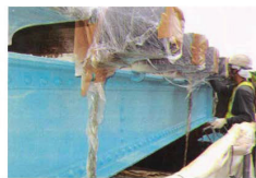
Shaded finish (blue color as example in above photo) can be applied as top coating for aesthetics purpose only, if required
