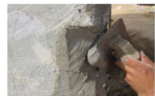
To fill repair material with spatula, trowel,
