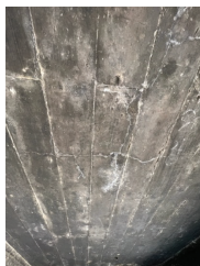
Cracks on the deck slab.
