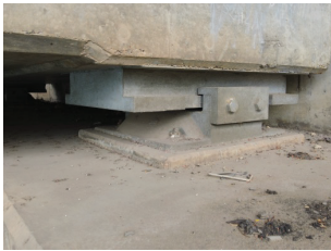
Sliding steel bearing used on Kilifi Bridge
