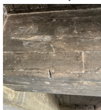
Rebar fractures and cracks on the main girder/cross beam.
