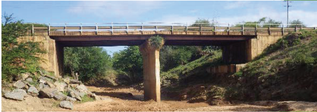
Simply supported bridge Nguutani Bridge along Thika - Garissa road
