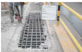
Removal of deteriorated deck slab
