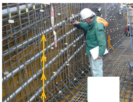
Before casting concrete
