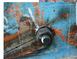
Bolt added to the hole
