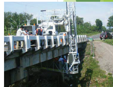
Access using an inspection vehicle
