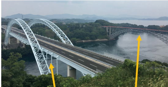
Left: Half-through bridge Right: Deck bridge
