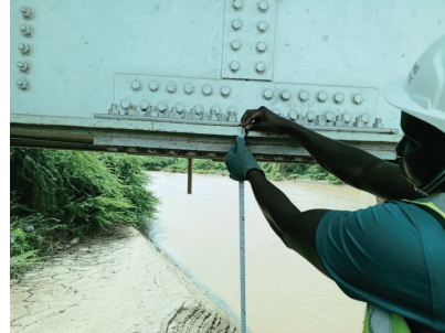
Bolted splice joint
