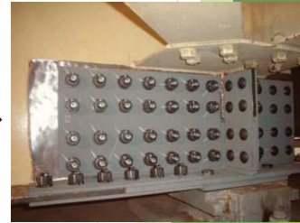
Steel plate added to the section.
