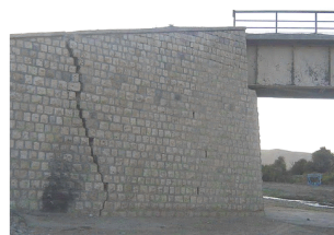
Cracks on the abutment/Retaining wall.
