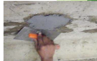
Placing mortar
