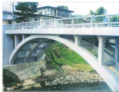
After Surface Sealing Work
