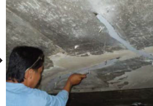
Drilling of holes and fixing injection pipes
