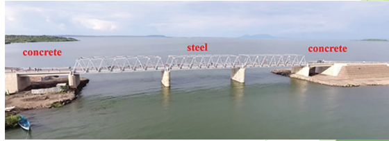
Composite material bridge
