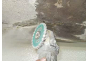
Preparing grooves for Caulking
