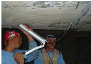
Injecting the Epoxy Grout
