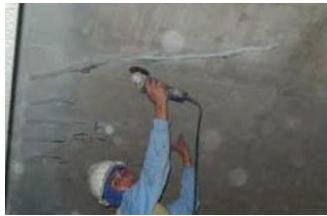
Cleaning Cracks
