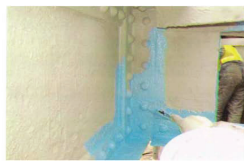
Shaded finish (blue color as example in above photo) can be applied as top coating for aesthetics purpose only, if required
