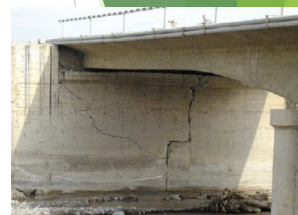
Cracks on the abutment/Retaining wall.
