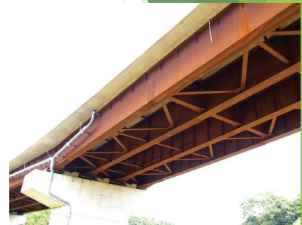
Corrosion protection on steel girders
