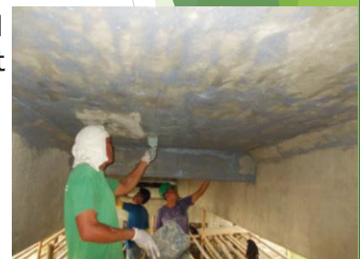
Application of protective coating
