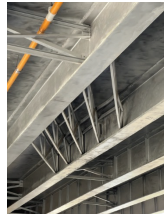
Deformation of steel girder/bracing.
