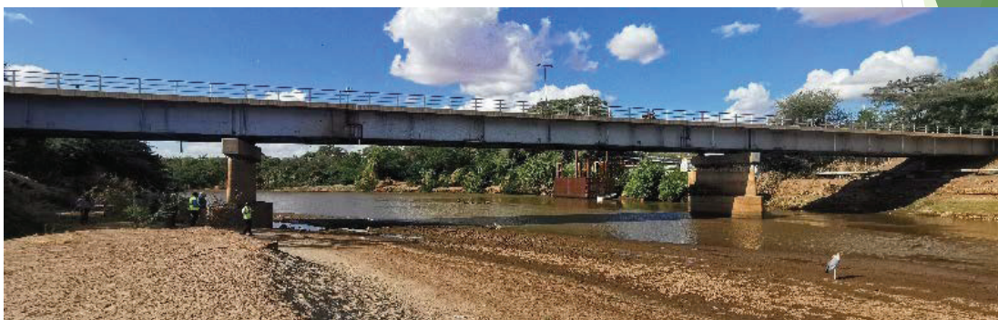
Cantilever/ Gerber Bridge Tana river bridge (Garissa) along A3
