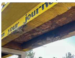
Rebar fractures and cracks on the main girder/cross beam.
