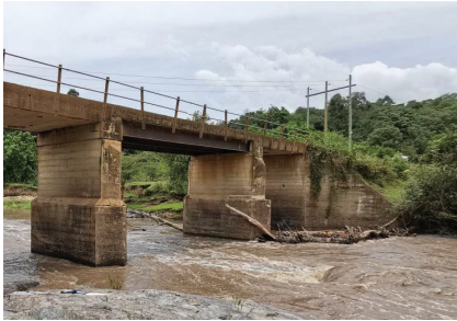
Accumulated driftwood obstructing the free flow of water.
