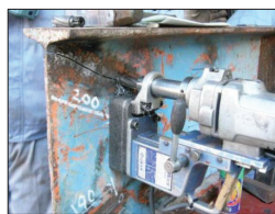
Drill stop hole
