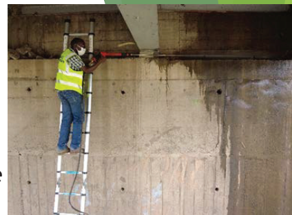
Cleaning using water pressure
