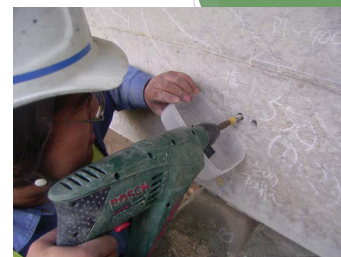
Drilling concrete
