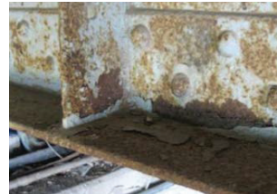
Corrosion of steel girder.
