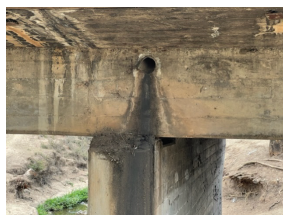
Siltation/Sedimentation on the bridge seat.
