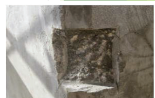
Preparation of repair section
