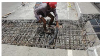
Placement of additional rebars and cleaning.
