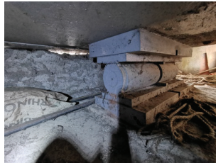
Roller steel bearing used on Nyali Bridge
