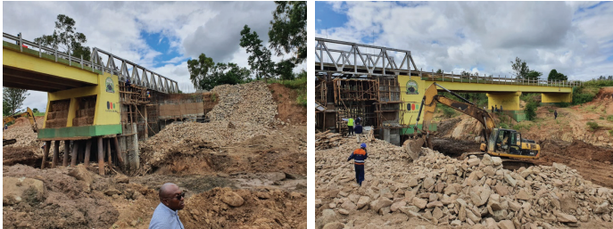
Pile repair works ongoing at Thwake Bridge
