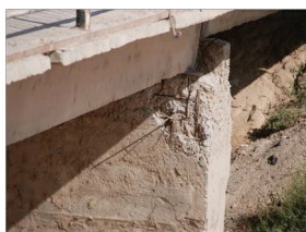
Sectional loss and rebar exposure of pier concrete.
