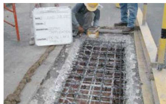
Preparation of old concrete and rebar and applying bonding agent
