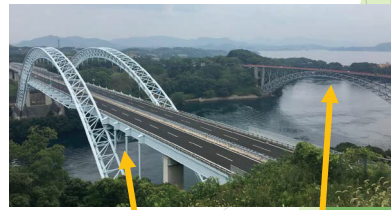
Left: Half-through bridge Right: Deck bridge
