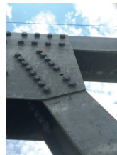
Missing and corrosion of bolts.
