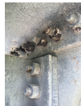
Missing and corrosion of bolts.
