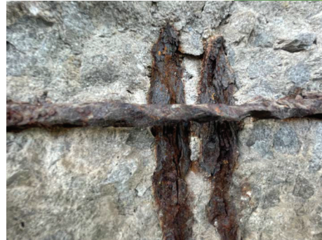
Nyali Bridge Abutment
