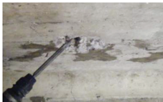
Removing loose particles
