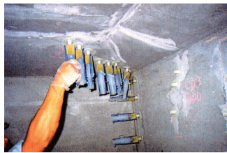
Epoxy injection work
