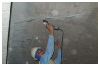
Curing of Injected Material
