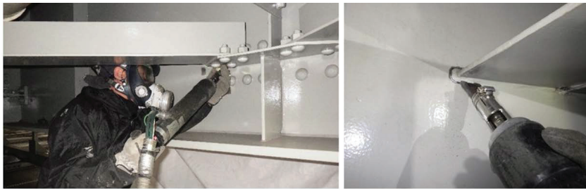
Welding in progress
