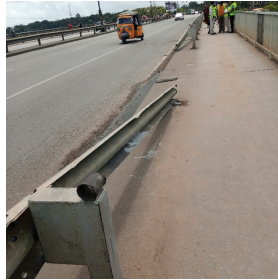
Damages on railings, guardrails, fences, and kerbs.
