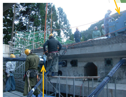
Tensioning work after the concrete hardens
