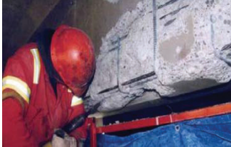
Removal of girder concrete.
