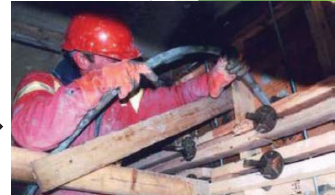
Grouting Mortar after setting formwork.
