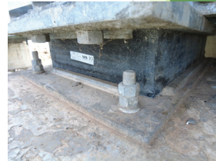
Elastomeric bearing used on Mbita Bridge
