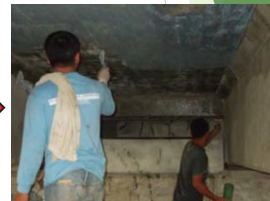
Applying mortar using trowel or brush.
