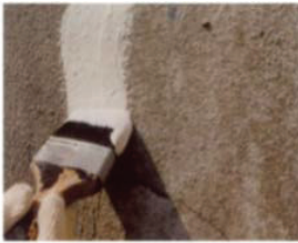
Surface sealing work
