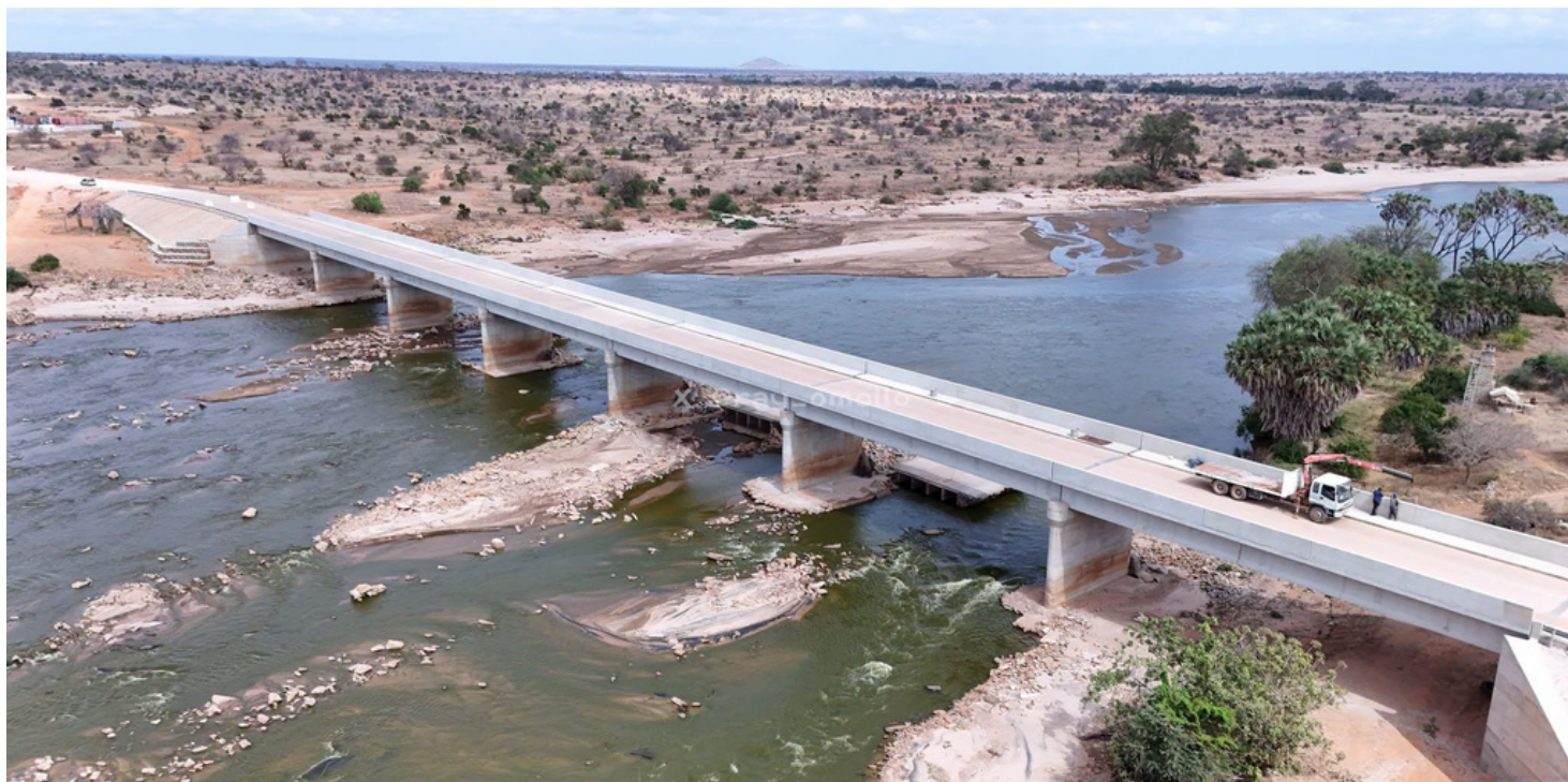
The new Galana–Kulalu Bridge
